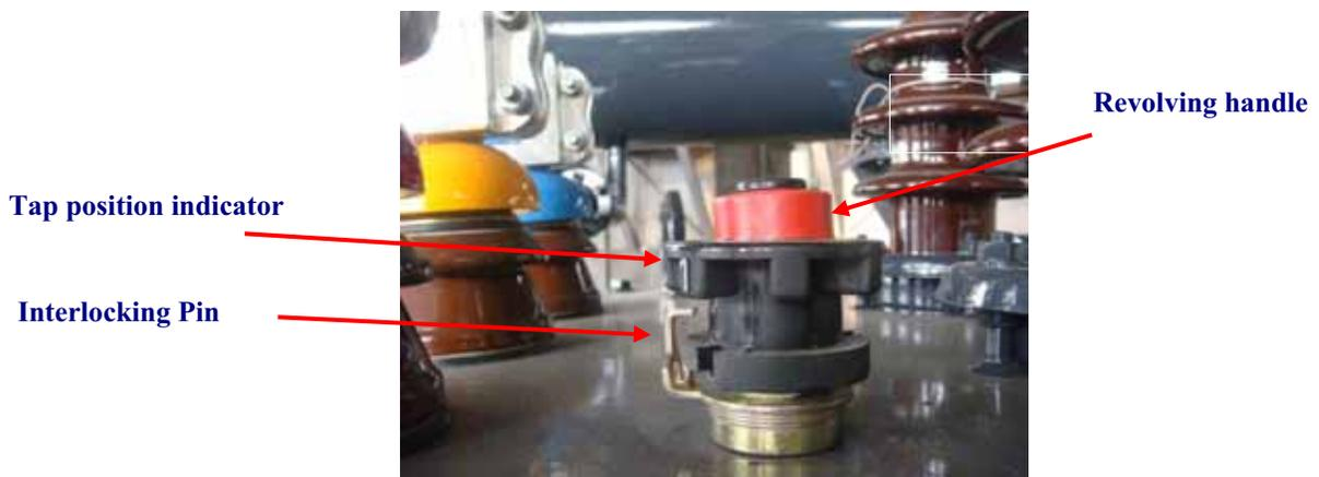
**Figure 11 : Different parts of tap changer**
