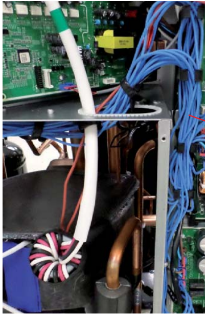
► Comp wire & valve,sensor wires fix by Holder wire with cover bushing hole.
