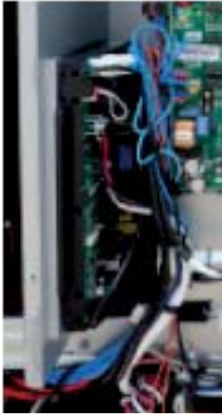
► Comp Wire fix by Holder Wire.
