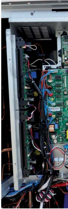
► Comp Wire fix by Holder Wire.
